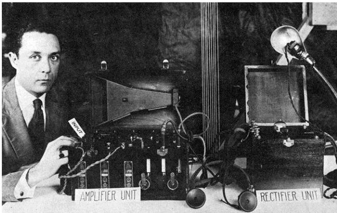
The “mousetrap” was a receiver for a radio amplifier that could run on AC. This was considered a breakthrough because at that time radios were only able to be powered by direct current (DC) provided by batteries. These batteries were bulky and heavy, had to be charged from time to time and were considered dangerous because of the acid used in them. The researchers’ prototype meant the radio could be used in homes without causing damage and with the same performance quality.
